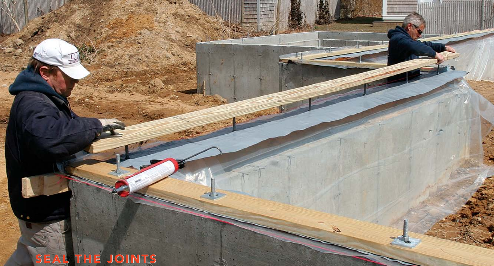
Butter the butt joints. Before placing the next 2x6 sill, a thick bead of sealant is applied to the edge of any adjoining sill. This is a commonly overlooked weak spot in an air-sealed assembly.
